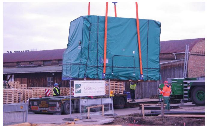
Delivery of the fuel cell module at the FRIATEC premises on 18 February 2016
